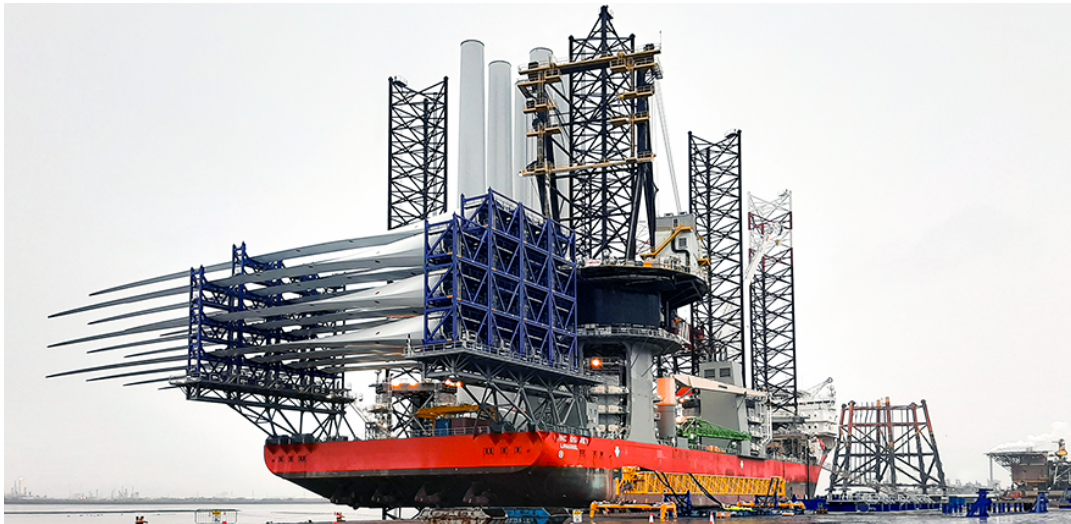
Figure 3.2: Blades stacked in a blade rack on an installation vessel
