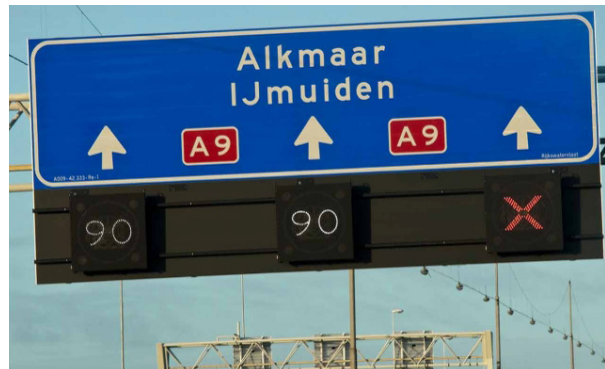
Figure 23: matrix signs showing the speed limit and a red cross (Plaatsengids, n.d.)
