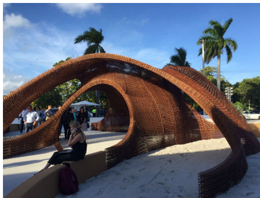
Flotsam&Jetsam, 255 sm, SHoP Architects Printed in 10 weeks, assembled in 4 days
