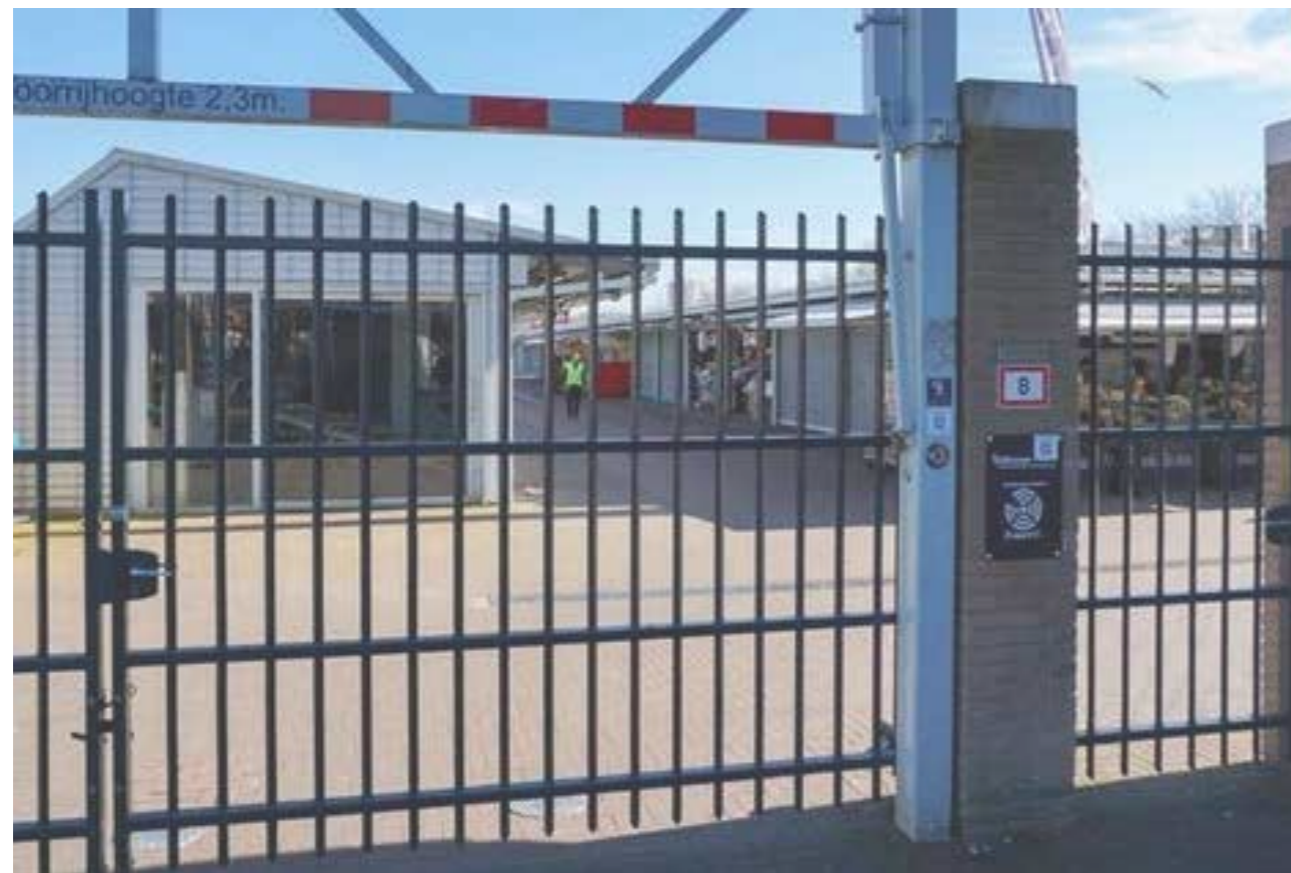
Fences on west side
