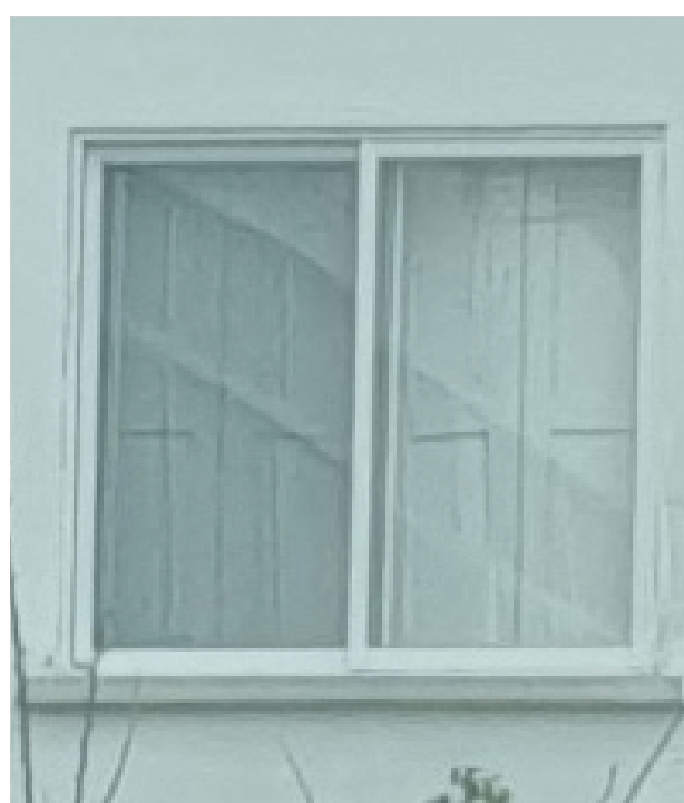
Replaced: PVC window frames (original wooden window frames)
