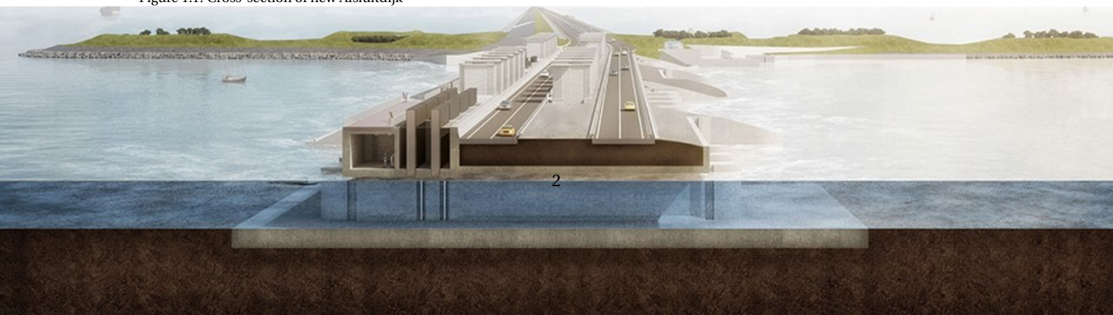
Figure 1.1: Cross-section of new Afsluitdijk
