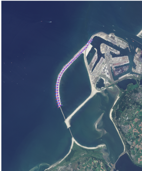
Figure 6.2: Visualisation of the connection and the location of each of the calculated rays, as represented in UNIBEST-CL (see Figure 6.1 and overlaid on the map of the research area).
