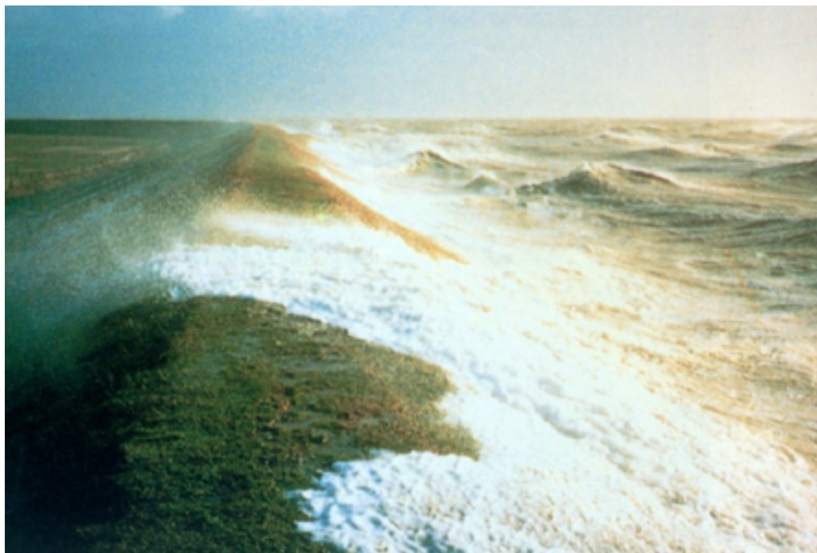
Figure 2.2: Photo of the overtopping of a sea dike at Hartepool, UK. Source: Flood Defences Lecture Notes, [7].
