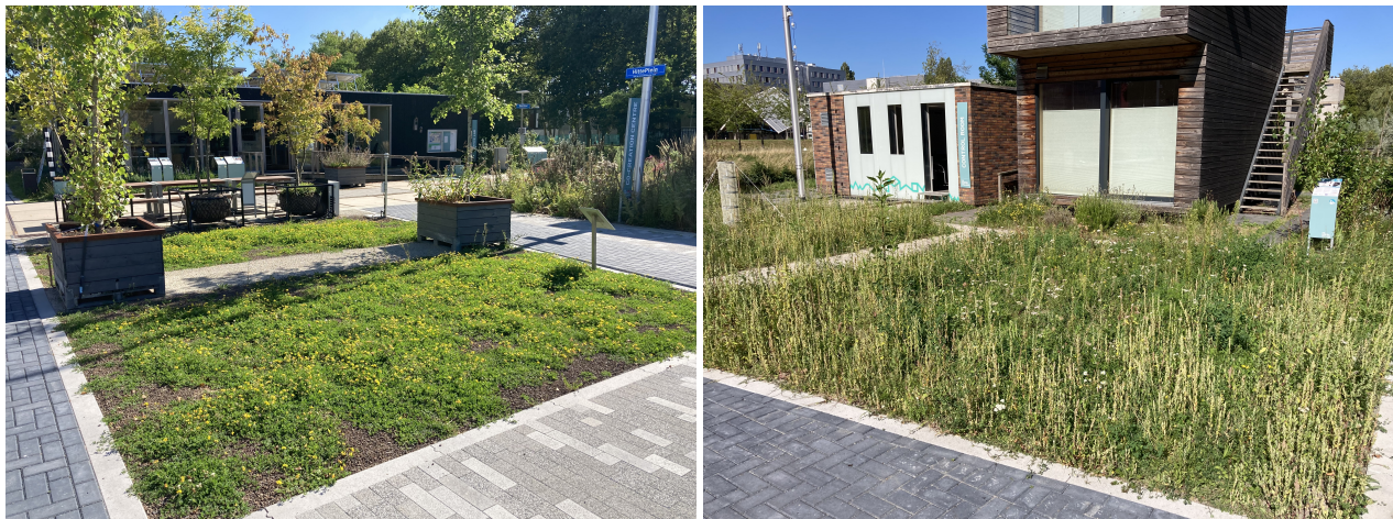
(a) Vegetation in 40 cm roof substrate.
