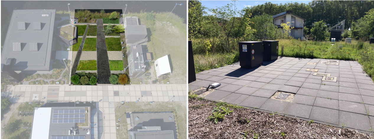
(a) Render of the renovated HeatSquare in The Green Village. (b) The Hydrogen Square in The Green Village.
