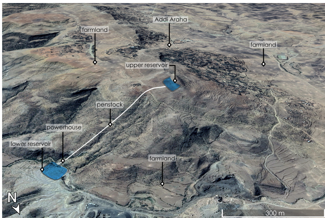
Figure 5.4: An overview of the suggested installation site for the PHS system. Obtained from Google Earth.
