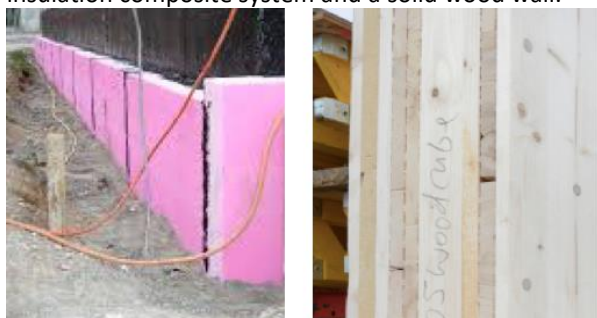
Figure 1: Wall with external thermal insulation composite system (left); solid wood wall (right)
