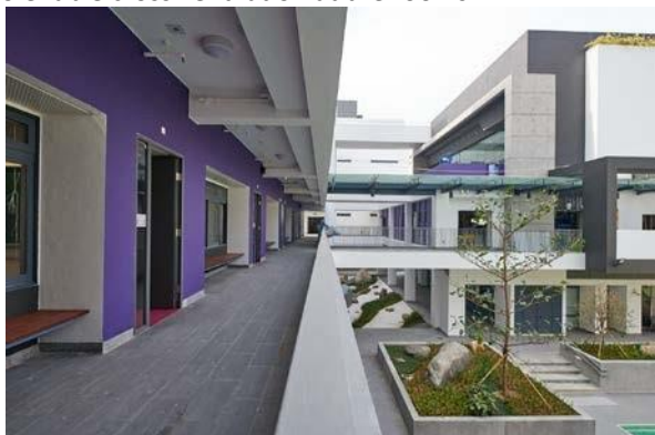
Figure 7: Open corridors with natural ventilation.
