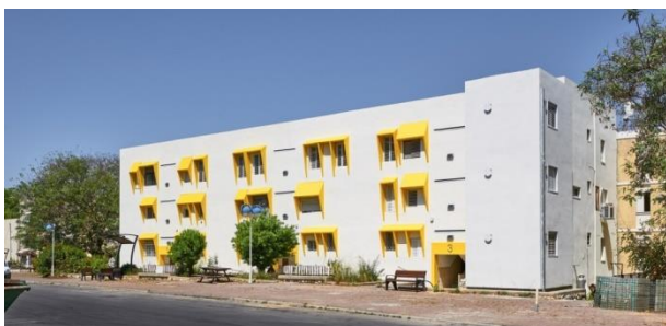
Figure 11: The south-west façade of the Sderot building after renovation: old windows with a uniformed shading system (photo: Lior Avitan)
