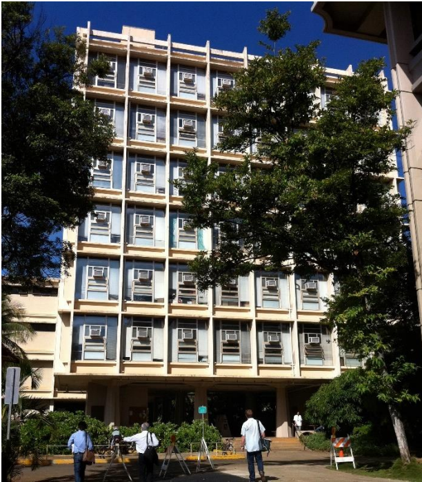
Figure 1: Exterior View of Kuykendall Hall Showing Window Air Conditioning Units in Professor Offices.
