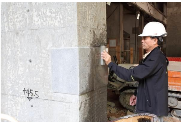
Figure 12: Experienced terrazzo artisans hand-trowelled terrazzo walls and floors.
