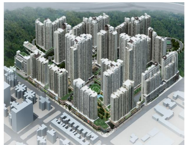
Figure 3: So Uk Estate
