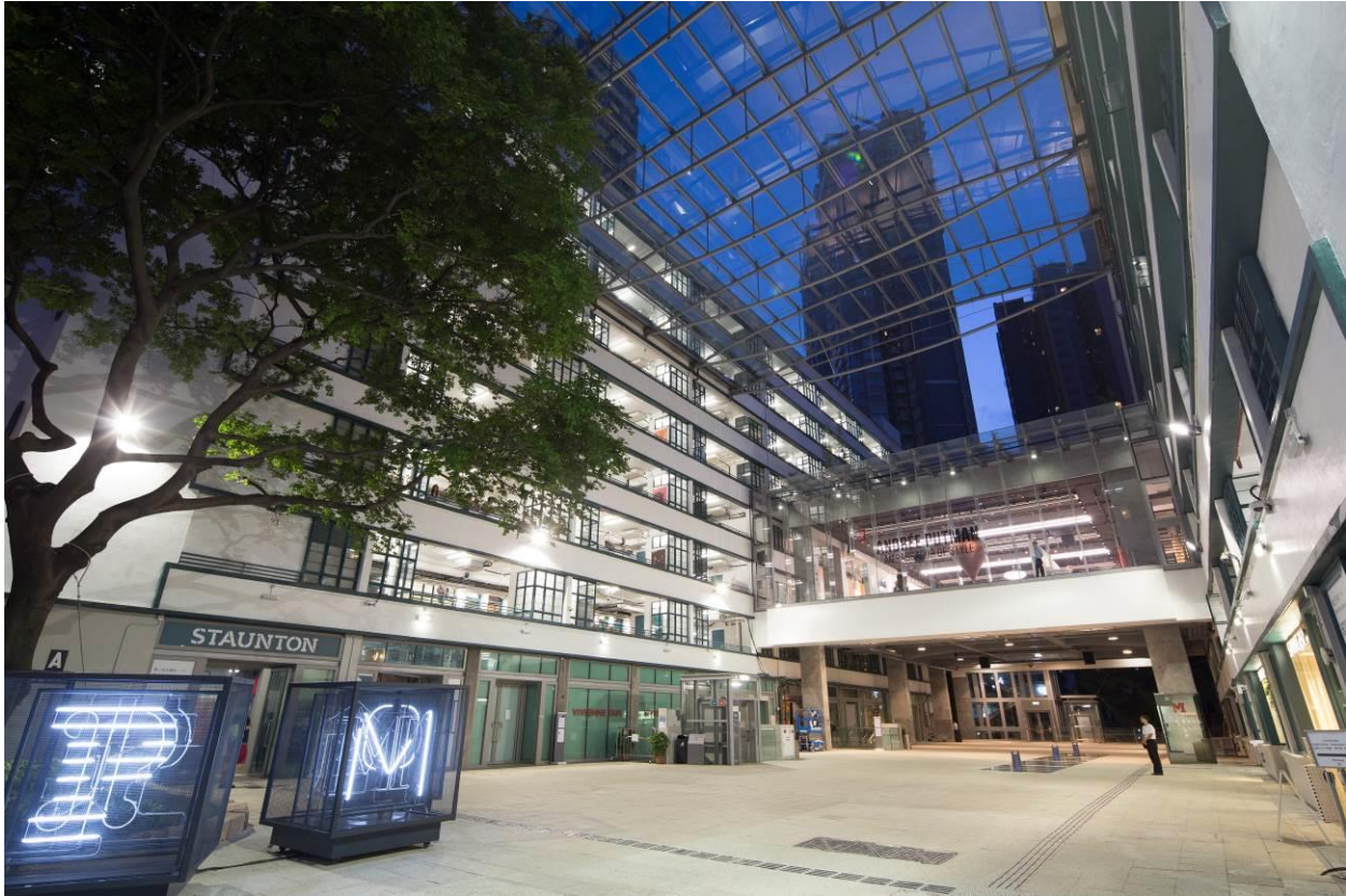
Figure 8: Precast steel truss members span across Block A and Block B to maintain a column-free courtyard.
