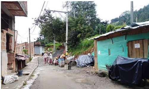
Figure 8: Improvement of the road in the Esfuerzos de Paz neighbourhood, Commune 8, Medellín
