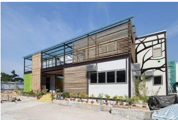
Figure 8: Green site office using second/third-hand construction materials.
