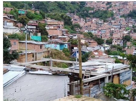
Figure 10: Housing in constructive process, Esfuerzos de Paz neighbourhood, Commune 8, Medellín.
