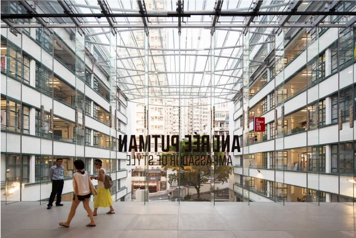
Figure 5: A view of the two Quarter Blocks through the crystal clear low-iron glass panels of the QUBE.
