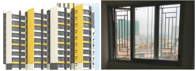
Figure 14: Vertical acoustic fins and acoustic windows were adopted to mitigate surrounding traffic noises according to the extent at respective locations.
