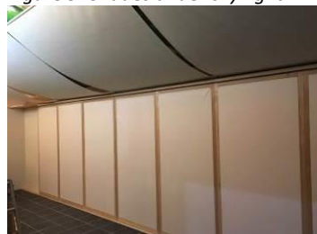
Figure 11: Windows systems installed inside windows for insulation.
