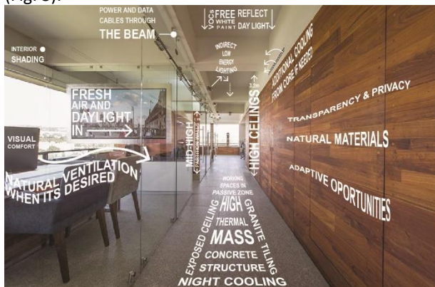
Figure 3: Photograph taken from the corridor of the analysed layout after the refurbishment - general construction details, passive strategies and design intentions are shown.
