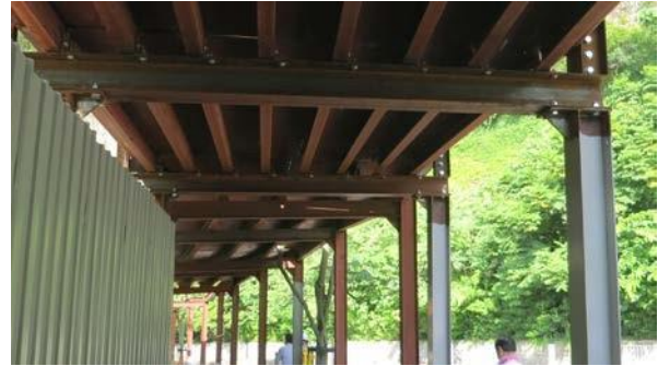
Figure 9: Bolt and nut hoarding – a reusable modular hoarding system.
