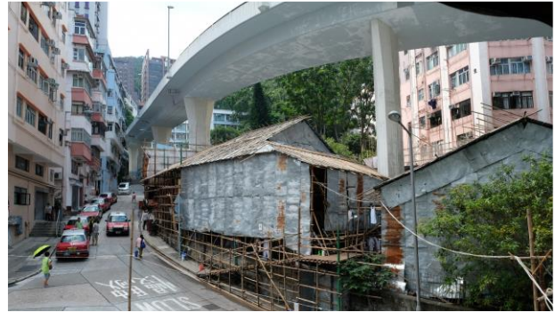
Figure 2: Hill Road Viaduct, Sai Ting Pun, Hong Kong. Photo P.W. Ferretto
