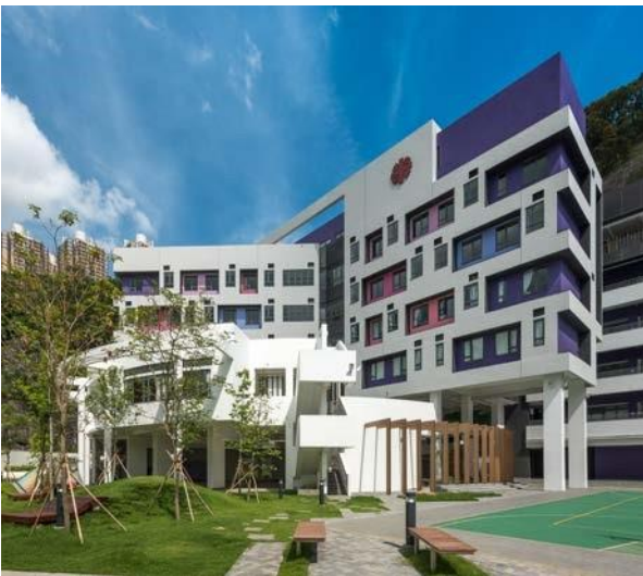
Figure 6: The external surfaces of the complex are largely painted in white – a low emissivity colour
