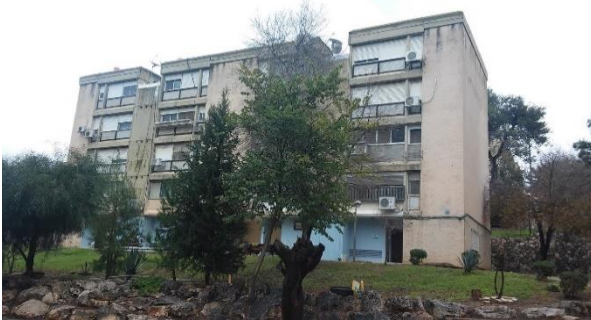
Figure 2: The Migdal Hahemek building before renovation, north-west entrance façade
