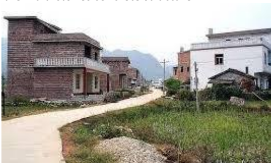
Figure 9: Concrete rural houses in China (Image from website)
