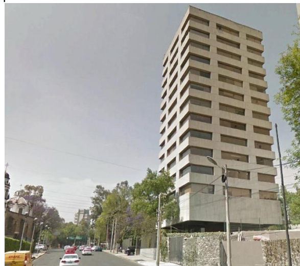
Figure 1: Canoa 521 building, Mexico City. On the right the concrete structure building which was analysed.
