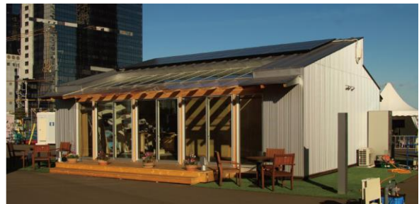
Figure 1: South facade of Kisekae House.
