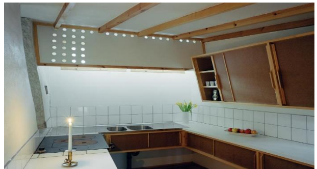
Figure 11: Indirect Lighting in the kitchen of Erskine House. The perforation of the upper panel allows to diffuse light and avoid contrasts.
