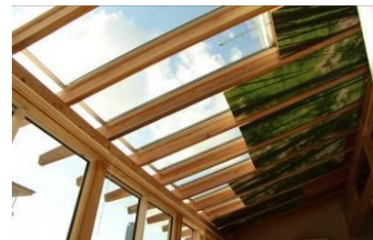
Figure 5: High-insulated shadings under skylights. They can be moved up and down manually and electric-powered.
