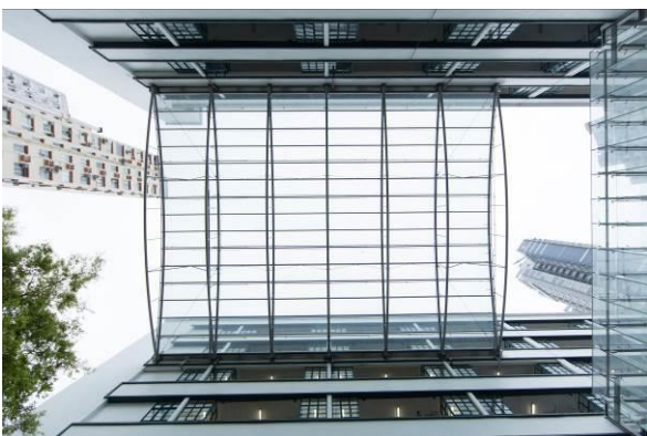
Figure 9: The Grand Canopy viewed from below.
