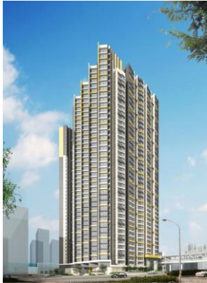
Figure 2: Subsided Sale Flats Development at FTSW
