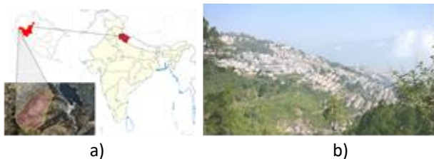
Figure 1: a) Location and b) Site View showing low-rise development in Tehri Township, Uttarakhand, India.
