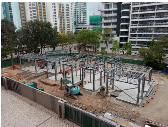
Figure 12: Steel frame erected during works.
