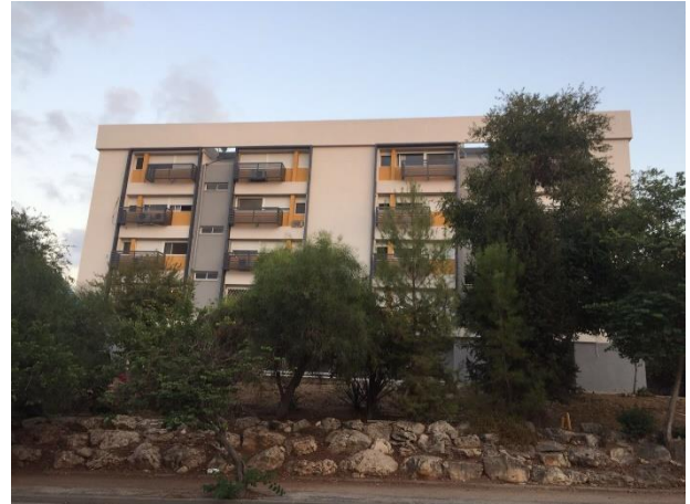
Figure 12: The north-west façade of the Migdal Hahemek building after renovation: new windows and roller shutters
