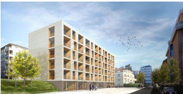
Figure 1: Architectural visualization of a BIPV scenario integrating CSEM's BIPV façade cladding. Base for the AAF demonstrator (Source: LAST).
