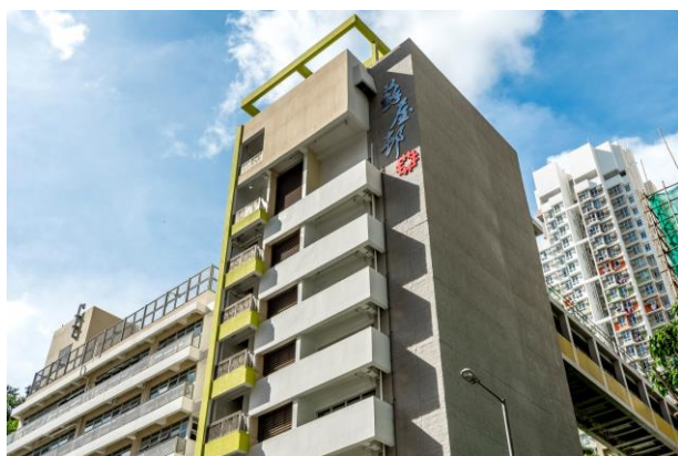
Figure 9: All building terraces are well connected with lift towers, escalators and footbridges. There are altogether 11 footbridges and 10 lift towers all subtly integrated with the buildings and the overall layout
