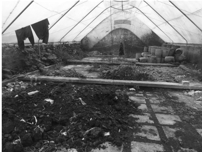
Figure 2: Solids handling, following dewatering at a community-scale FSTP in Kanyama neighborhood Lusaka, Zambia. (Picture by Nienke Andriessen)
