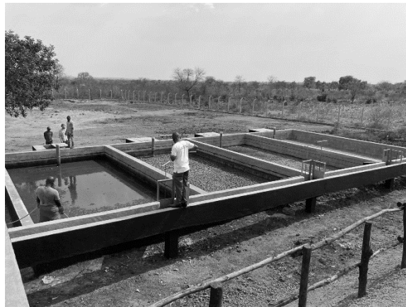
Figure 5: Waste stabilization ponds from the Imvepi FSTP in Uganda. (Picture by Nienke Andriessen)
