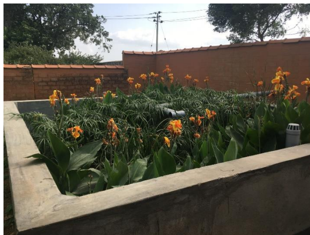
Figure 6: A planted drying bed from a small FSTP in Bangalore. (Picture by Nienke Andriessen)
