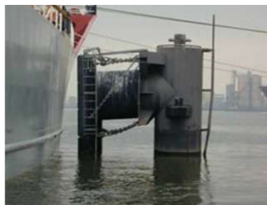
(a) Breasting dolphin
