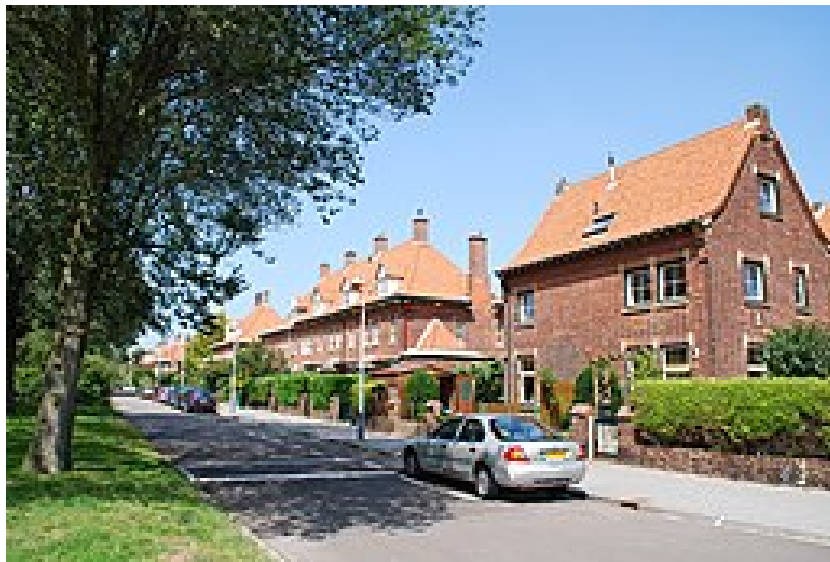
Figure B.9: Ensemble of houses in the Vogelwijk
