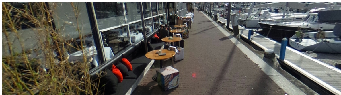
Figure 8.7: The current configuration of a part of the Doctor Lelykade. One can obviously see how a construction on top of the current quay wall would impose problems for stakeholders making use of the quay wall. The small black boxes indicate the/a physical boundary between the driving lanes. This is however a small part of the area. (Google Street View)
