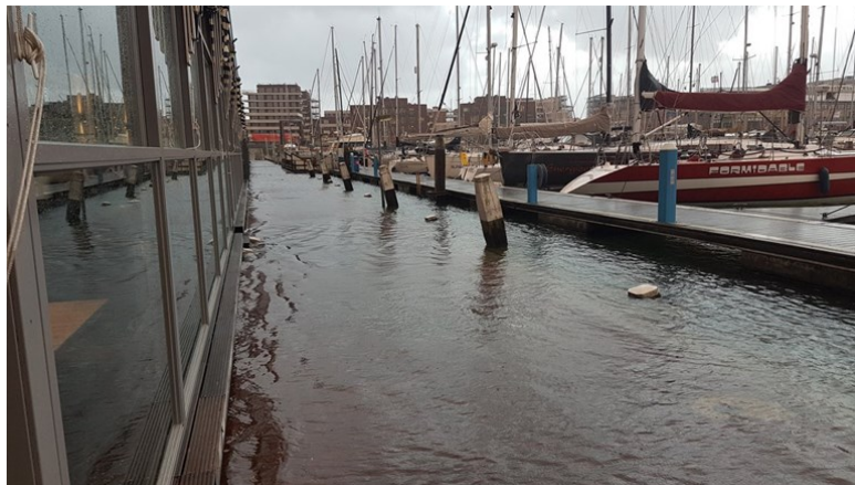
Figure 1.1: Flooding of the second harbour (Source: Omroepwest 2019)
