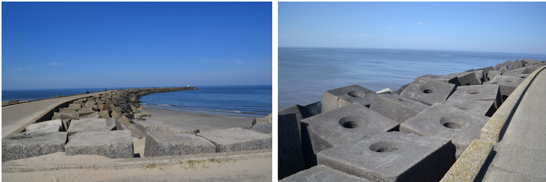
Figure 9.2: Currently the breakwaters are build with two types of concrete armour blocks.
