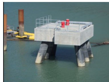
(b) Mooring dolphin
