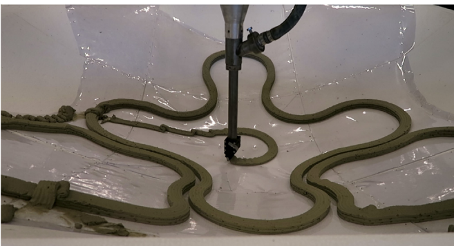
Fig. 20. Printing of final pavilion.
