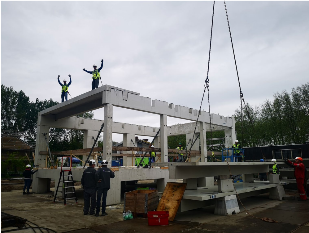
Assembly of the prototype's concrete structure _ MOR Team TU Delft
