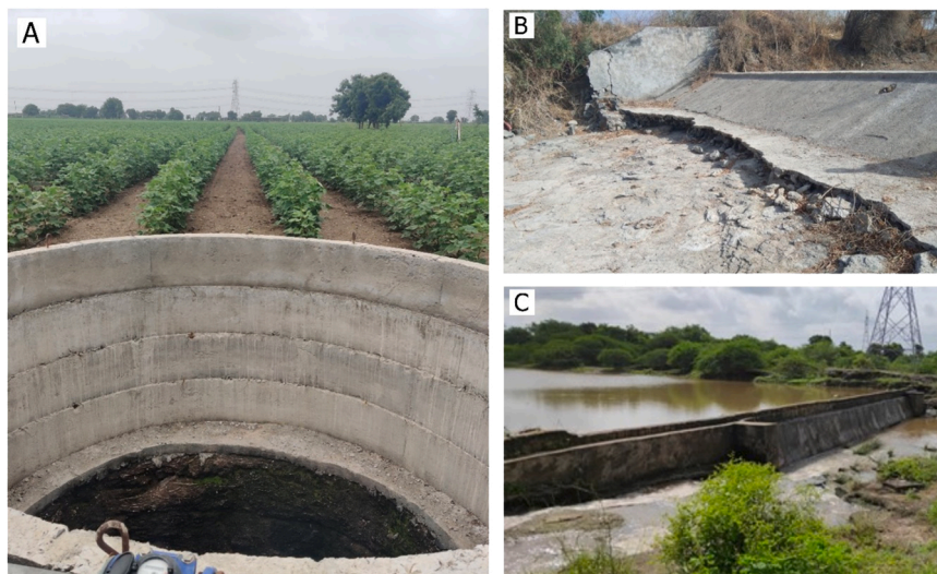
Fig. 2. a) Open dugwell commonly used for irrigation in the Bhadar basin; b) and c) check dam in the area in dry and wet season, respectively (images taken from downstream side).
