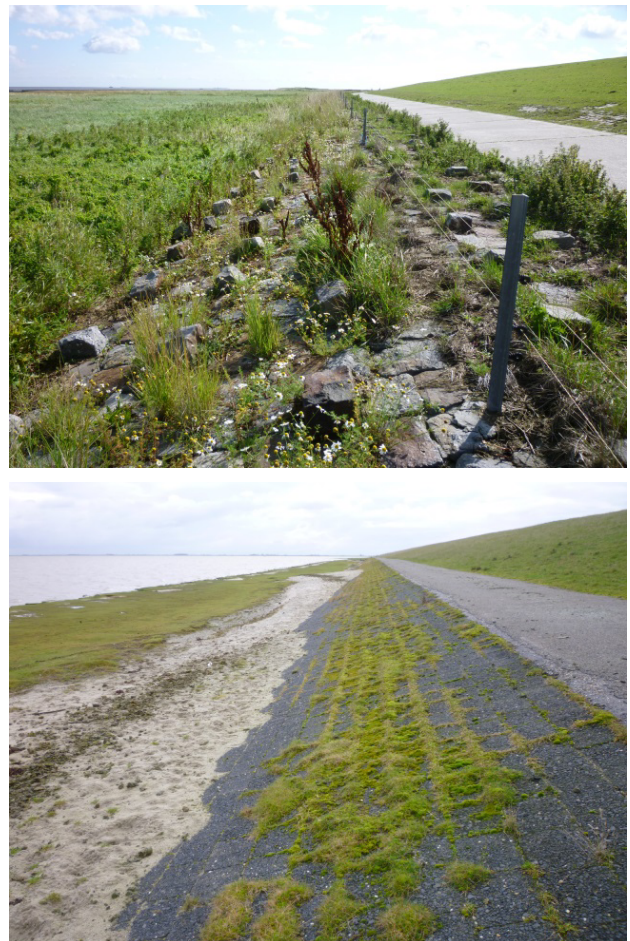
Figure 2: Dike with an adjacent broad salt-marsh zone (Elisabethgroden, Germany, top) and dike with a narrow salt-marsh zone (Dollard, Netherlands, bottom).
