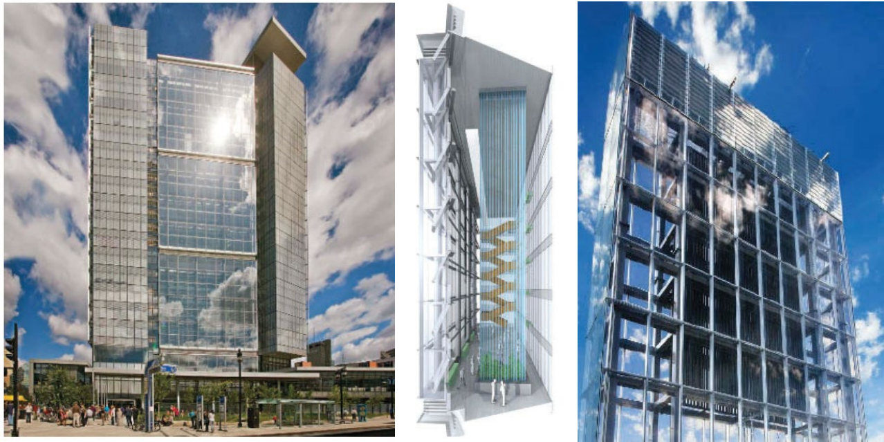
Figure 30 Left to right: Manitoba Hydro Place's South Façade, water feature, the top of the solar chimney (Wood & Salib, 2008)
