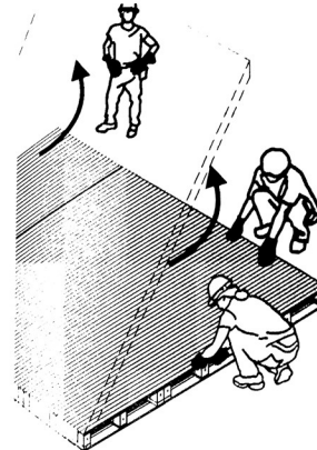
5. The walls are put up and placed in their new site.
