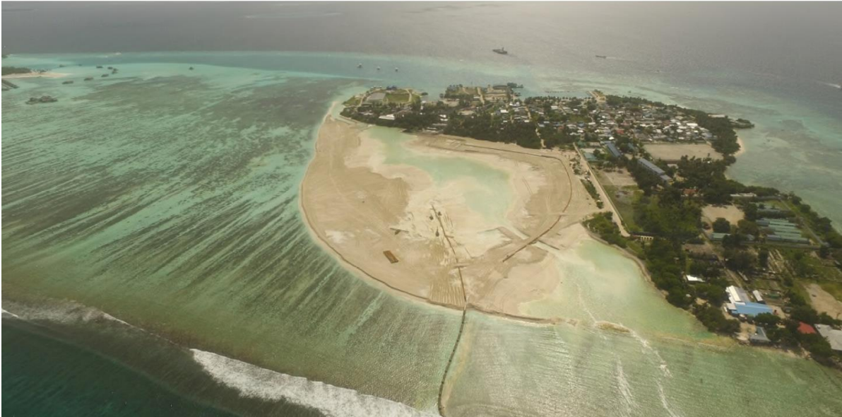
Figure 23 - Drone picture of reclamation works at Himmafushi - (Van Oord, 2017a)
