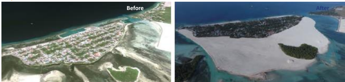
Figure 17 – Aerial images of the four project site before (left) and after project completion (right) – (Van Oord, 2017a)
