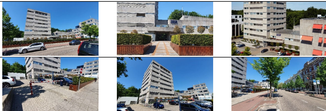
Figure 152: Pictures of the building along Bezuidenhoutseweg 60 (Vastgoeddata, 2023)
