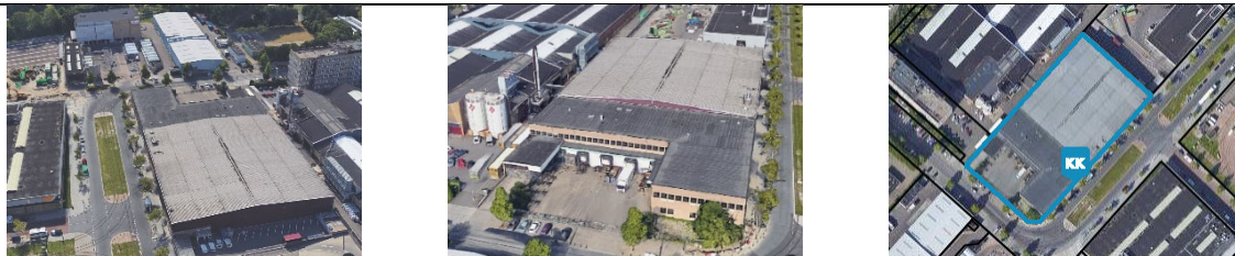
Figure 197: Aerial view of De Werf 13 and plot of De Werf 13 (Google Earth, N.D.; Kadastrale kaart, N.D.)
