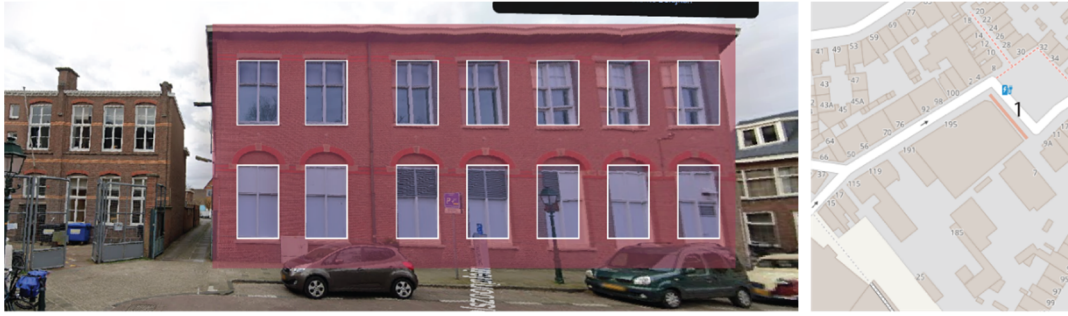
Facade 1 | Approximately 31% of facade is glass.
