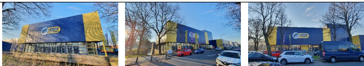
Figure 115: The main entrance of the building, which is the only part of the building with a significant amount of windows; the rest of the building is completely closed off and clad with blue panelling (Vastgoeddata, 2023)
