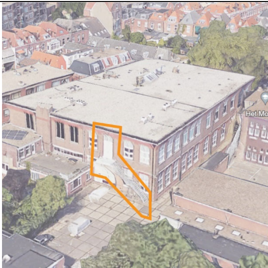
Figure 142: External staircase leading to the inner yard of the building along the Kerklaan 195 Open Street Map (N.D.)
