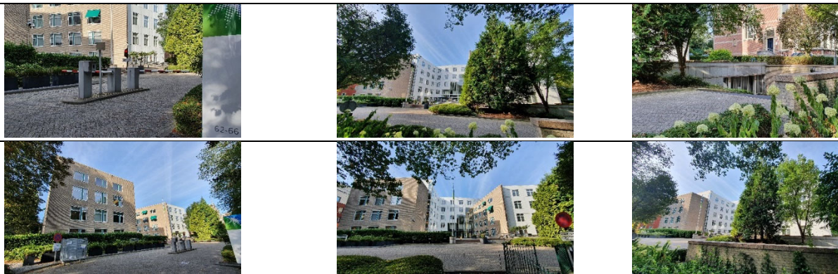
Figure 108: Selection of pictures of the building along the Scheveningseweg 64 showing the entrance by car past the gate up to the ramp that goes to the underground car parking lot (pictures 1, 2 and 3) and the front side of the building (picture 4,5 and 6)(Vastgoeddata, 2023)
