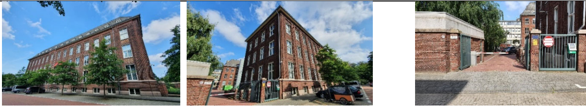
Figure 190: Pictures of the building along the Oostduinlaan 2 showing the left side of the façade along the Emantsstraat (picture 1), the entrance to the parking lot from the Emantsstraat (pictures 2 and 3) (Vastgoeddata, 2023)
