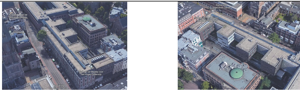
Figure 185: Aerial view of Oranjestraat 15 (Google Earth, N.D.)
