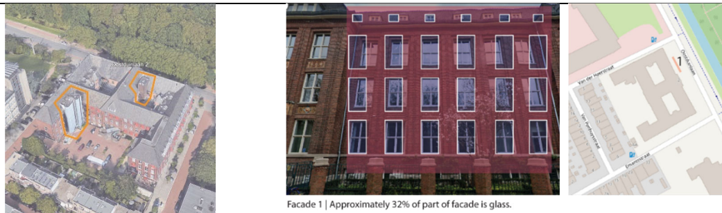
Figure 192: The shafts for the external staircases/lifts (picture 1) and the rhythm of windows in the façade of Oostduinlaan 2 (own image)
