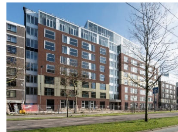
Figure 11: Transformation of DCMR building in Schiedam into apartments (Van Wijnen, N.D.-b)
