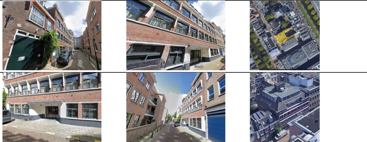
Figure 207: Pictures of the back side of the building along the Prinsessegracht 21 (Google Earth, N.D.)
