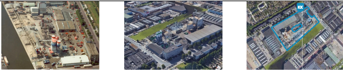
Figure 127: Zonweg 33 (1975) showing the office building on the right, aerial view of Zonweg 33 and plot of Zonweg 33 (Google Earth, N.D.; Kadastrale kaart, N.D.; Stichting Haags Industrieel Erfgoed, N.D.-b)
