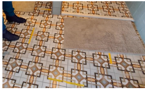
Fig. 6. Ella's bathroom floor markings indicate where the floor gets warm and where it does not.
