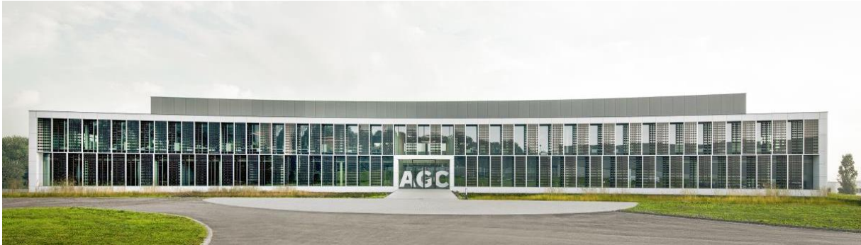
Figure 45 Front view of the case study building (Assar Architects, 2017)
