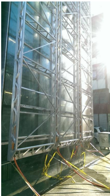
Figure 40 On-site water-tightness testing (gpf-innovation.ch)
