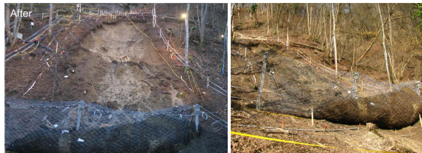
Fig. 13: Photographs of the Ruedlingen slope sediment after the debris flow of 17 March 2009. Note the deformation of the debris that accumulated in front of the barrier. Reproduced from [3].
