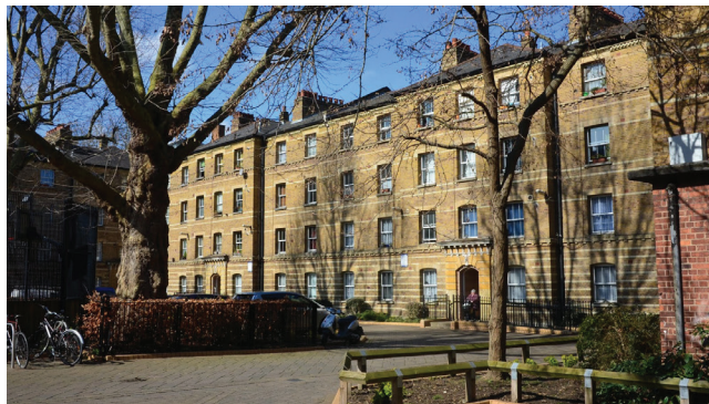
Figure 1.1 (clockwise from top) Peabody Square estate, overview, entrance and central courtyard
