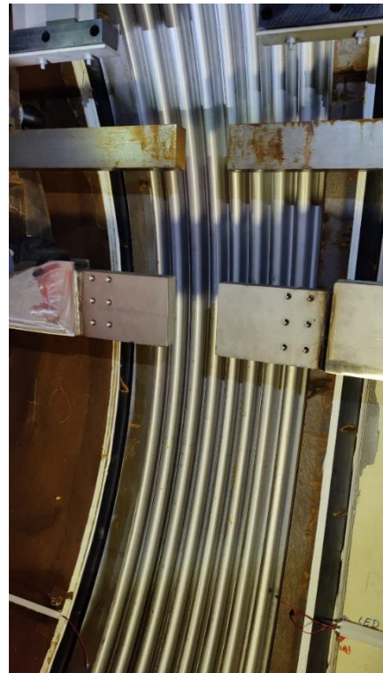
Figure 10: Expansion joint from the inside of the tube
