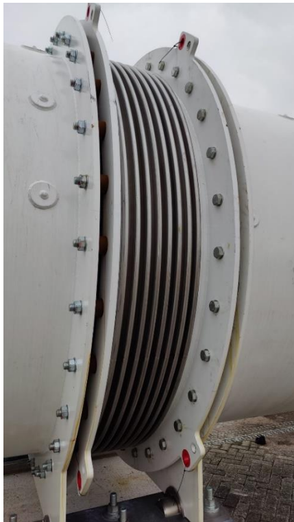
Figure 9: Expansion joint from the outside of the tube
