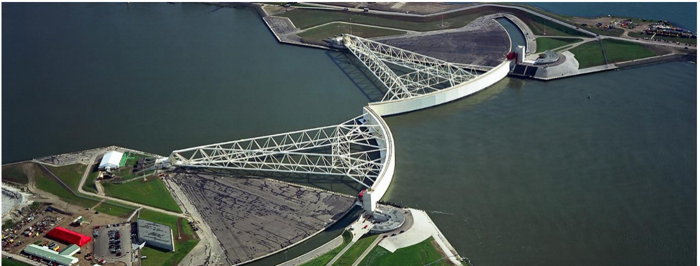
Figure 2: The Maeslantbarrier. The retaining walls are the large curved white element at the (in the picture) most right side of the Maeslantbarrier.
