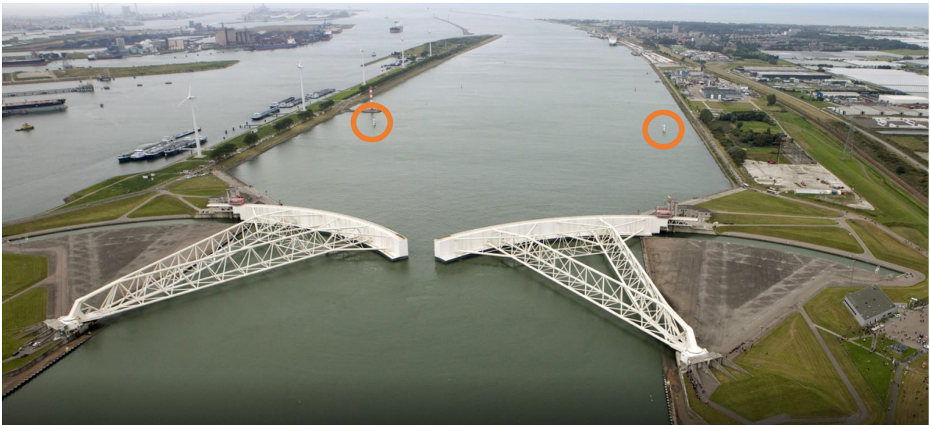
Figure 48: The Maeslant barrier with the water level measurement locations on the seaside of the barrier indicated in orange. These measurement stations are located downstream of the barrier. There are two more locations where the water level is measured, these are more upstream of the barrier, not visible in this figure.
