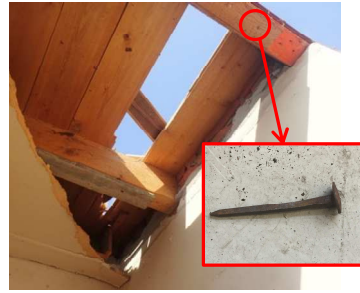
(b) connections between planks and timber joist
