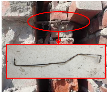
(a) three leaves interconnected with ties
