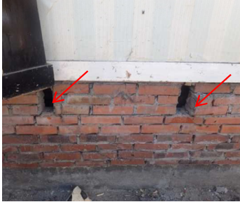
(c) joist pockets
