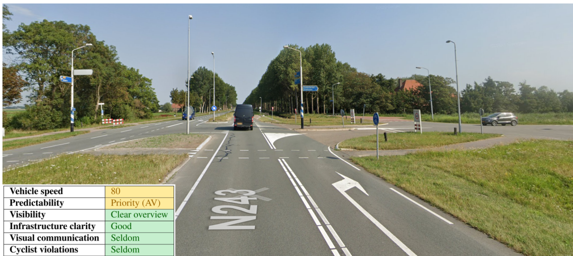
Figure 6.1: Example of a conflict situation with minor cyclist safety risks (N243 #1)
