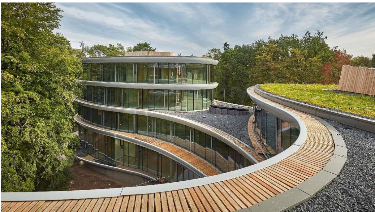
Figure 13 -Triodos Bank view from the roof, picture taken (Architectweb, 2019).
