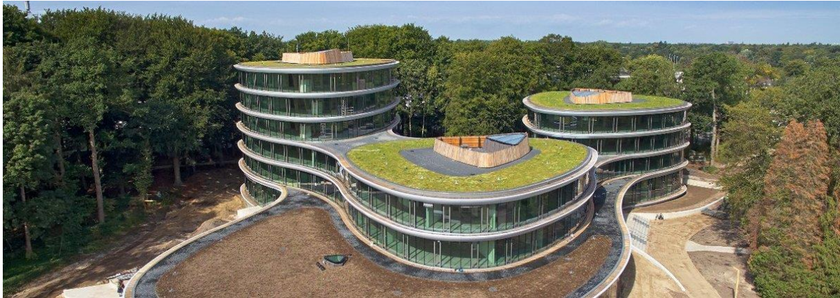
Figure 16 - Helicopter view Triodos Head office (Architectweb, 2019).
