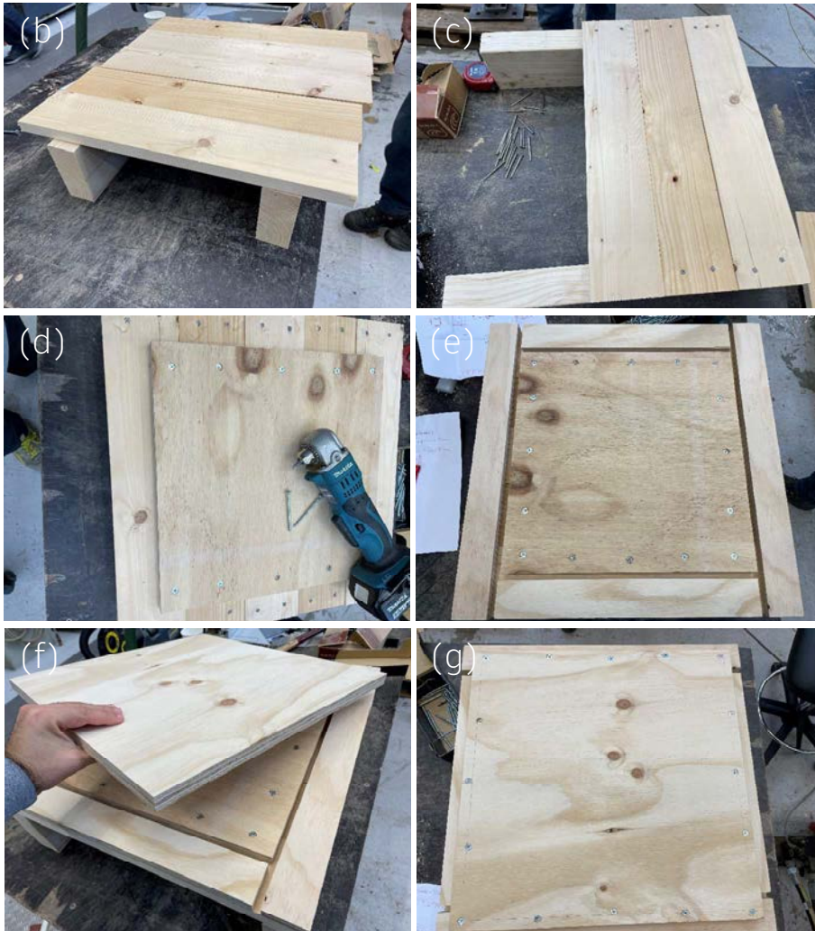
Figure 2: (a) Geometry and dimensions (in mm) of the tested prototype and construction sequence: (b) preparing joists and boards; (c) nailing the planks; (d) fastening the first plywood panel; (e) preparing the interlayer with plywood boards; (f) placing the second plywood panel; (g) fastening the second plywood panel.
