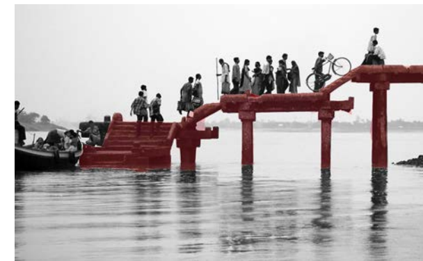
Figure 68: Improper Jetty Infrastructure (Source : Sightsavers, 2017) https://www.sightsavers.org/from-the-field , Edited by Author)
