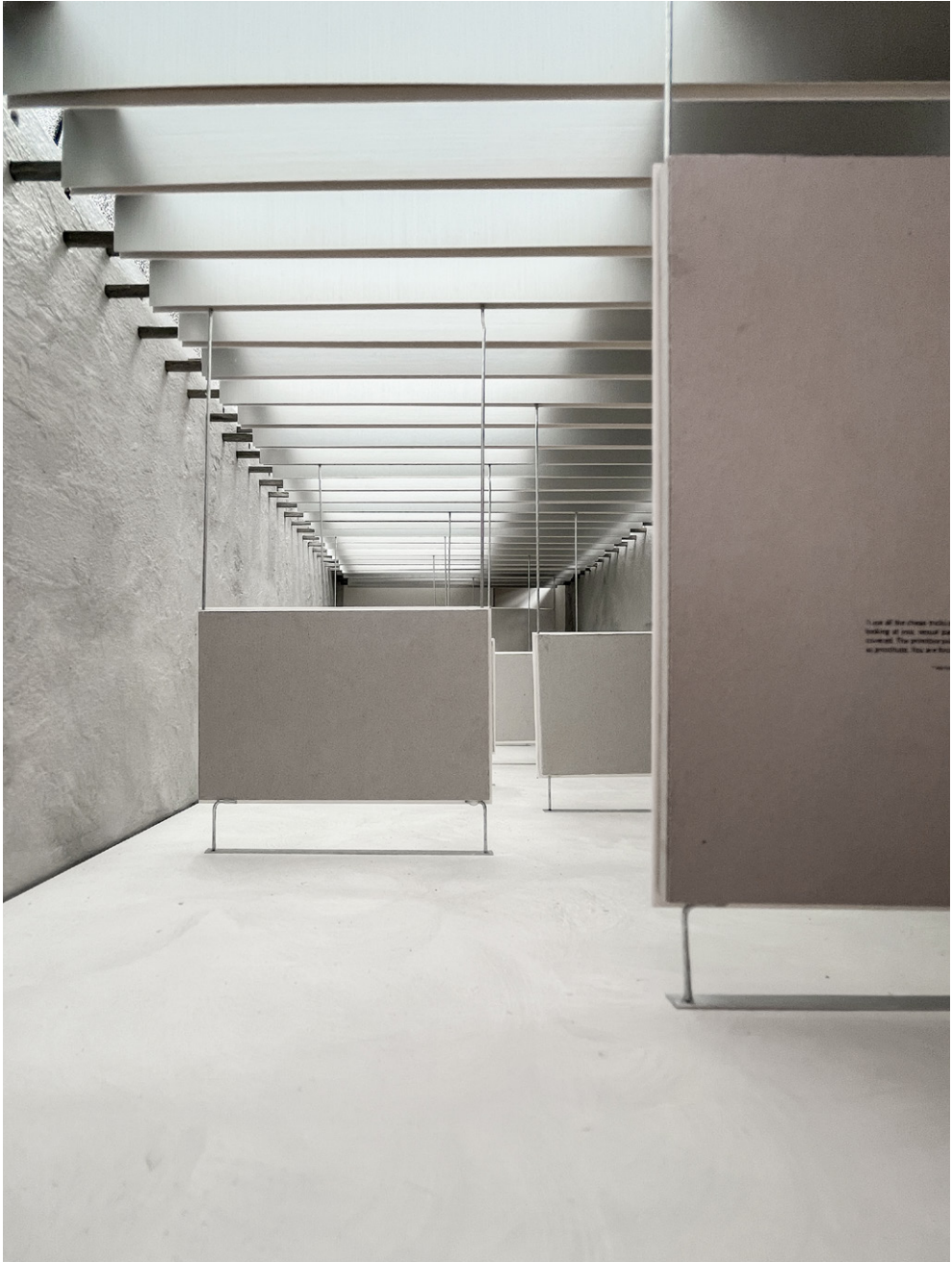
Picture of Model for Mariene Dumas showing the walls attached to the beams.
