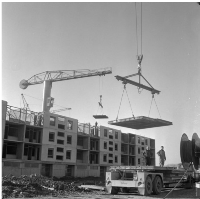
Fig 8. Cranes transporting prefabricated panels at the building site (Dura B.V., n.d.)
