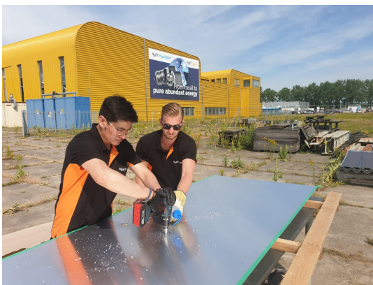
(a) Drilling the holes.
