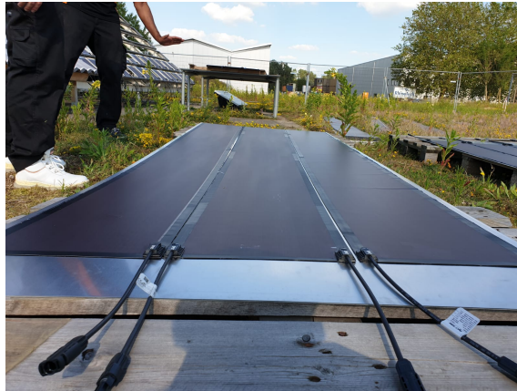
(b) Sticking the modules in place.
