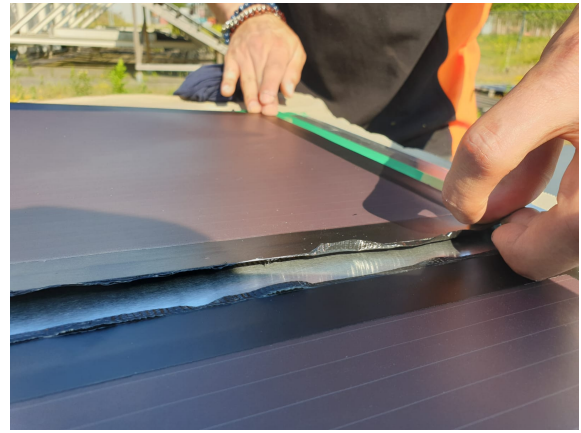
(b) Sticking the modules in place.
