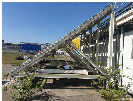
(b) Lateral view of structure
