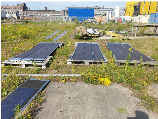
(a) Plates before installation.
