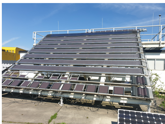
(a) Front view of structure
