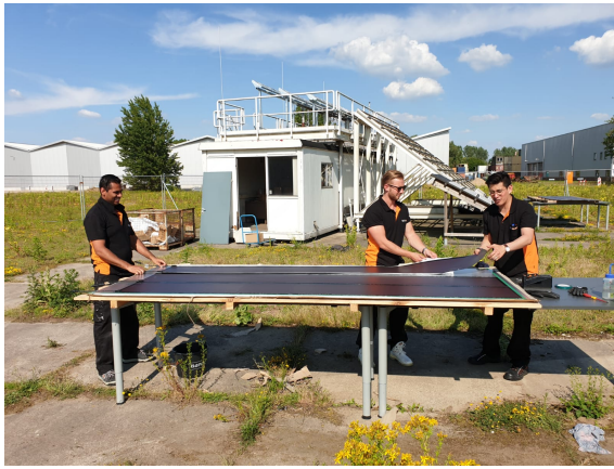
(a) Placing the modules.
