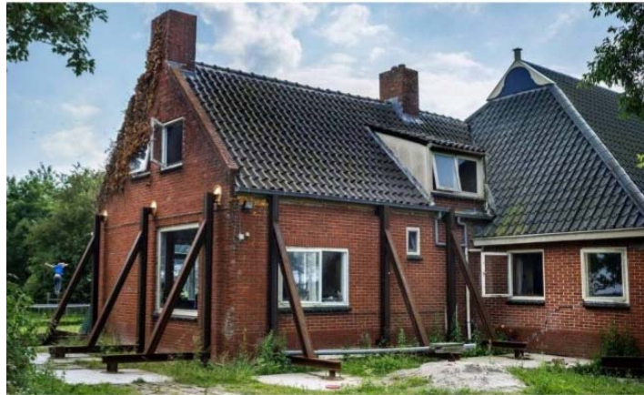
Figure 1 - A measure for collapse prevention in Loppersum.
