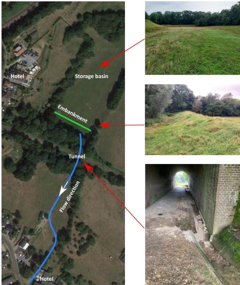
Figure 13: Location of Ransdaal storage basin near Schin op Geul (left) and images of the basin, the dike/embankment, and the erosion in the tunnel downstream (photographs provided by Bas Jonkman, TU Delft).
