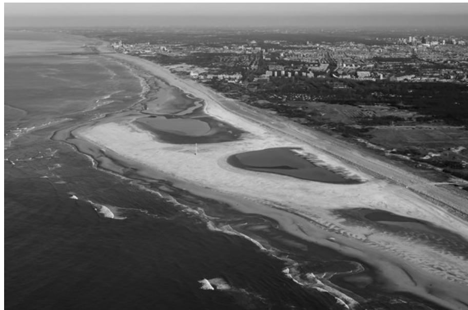
Illustration 1: The Sand Engine mega-nourishment seen from the South-West (Rijkswaterstaat) [6]
