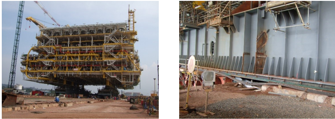
Figure 2.4: McDermott Load-Out Beams (McDermott)
