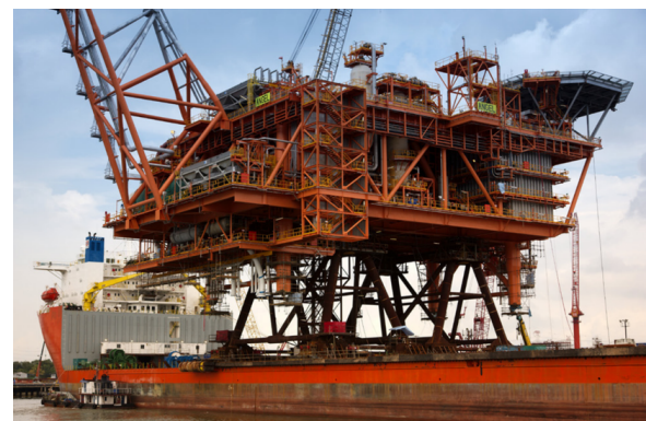
(b) Full construction (Angel)
