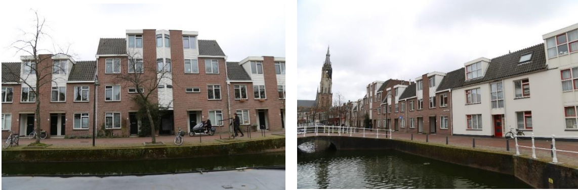
Figure 42: Pictures of the building (own work)
