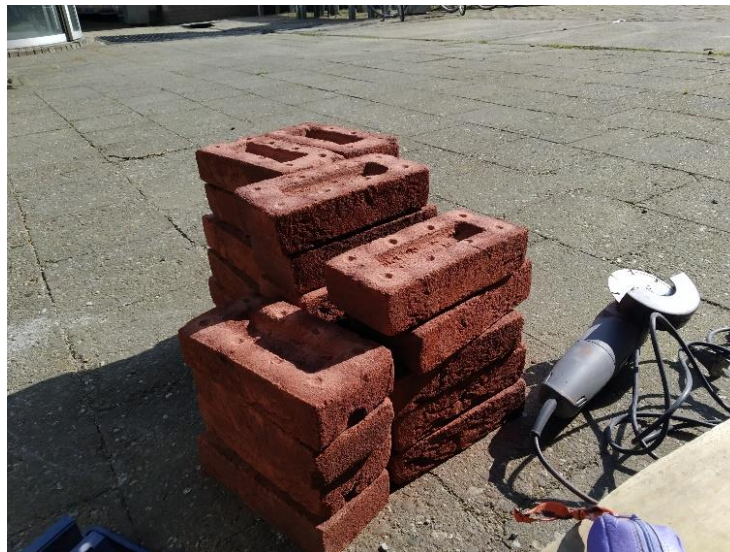
Figure 74: Drilled bricks (own work)
