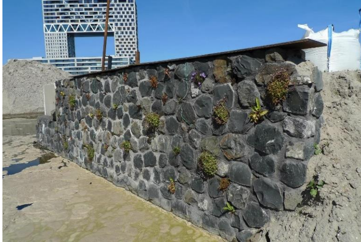
Figure 25: Mock-up quay wall (Ton Denters et al. 2019, 'Foto's d.d. 13-05-2019')
