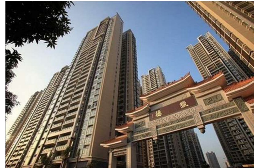
Figure 17. Market-led redevelopment project in Liede village, Guangzhou city, China (Source: SohuNews (2019), https://www.sohu.com/a/344468189_692677 , [retrieved on Nov 12, 2020])
