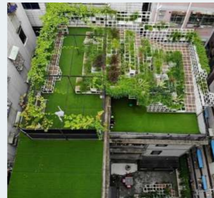
Figure 102. Roof garden in Shenzhen urban village.
