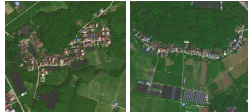
Figure 49. Traditional villages in Guangzhou suburban areas (Source: Baidu Map, https://map.baidu.com/ , edited by author)
