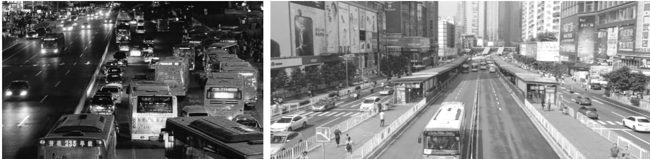
Figure 74. Shipai east road (left) (Source: https://www.163.com/news/article/58K9367A000120GR.html ); Tianhe road (right) (Source: SohuNews (2018), https://www.sohu.com/a/256478406_99997541 )
