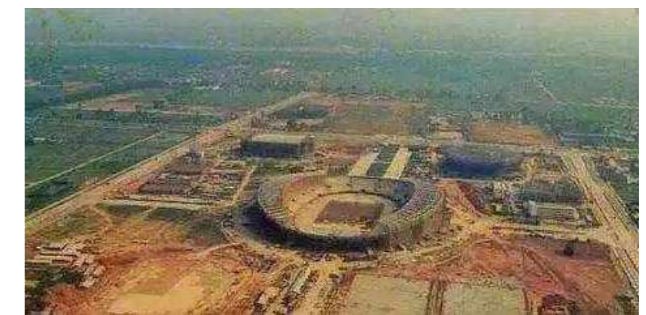
Figure 61. Construction of Tianhe sports center and railway station in 1987 (Source: https://www.sh-gongxin.com/kejixinwen/22550.html )
