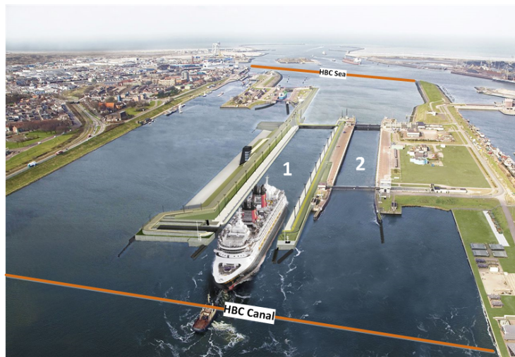
Figure F.1: Hydraulic boundary condition simplification for multiple navigation lock chambers in a complex (source: Beeldbank RWS, edited)
