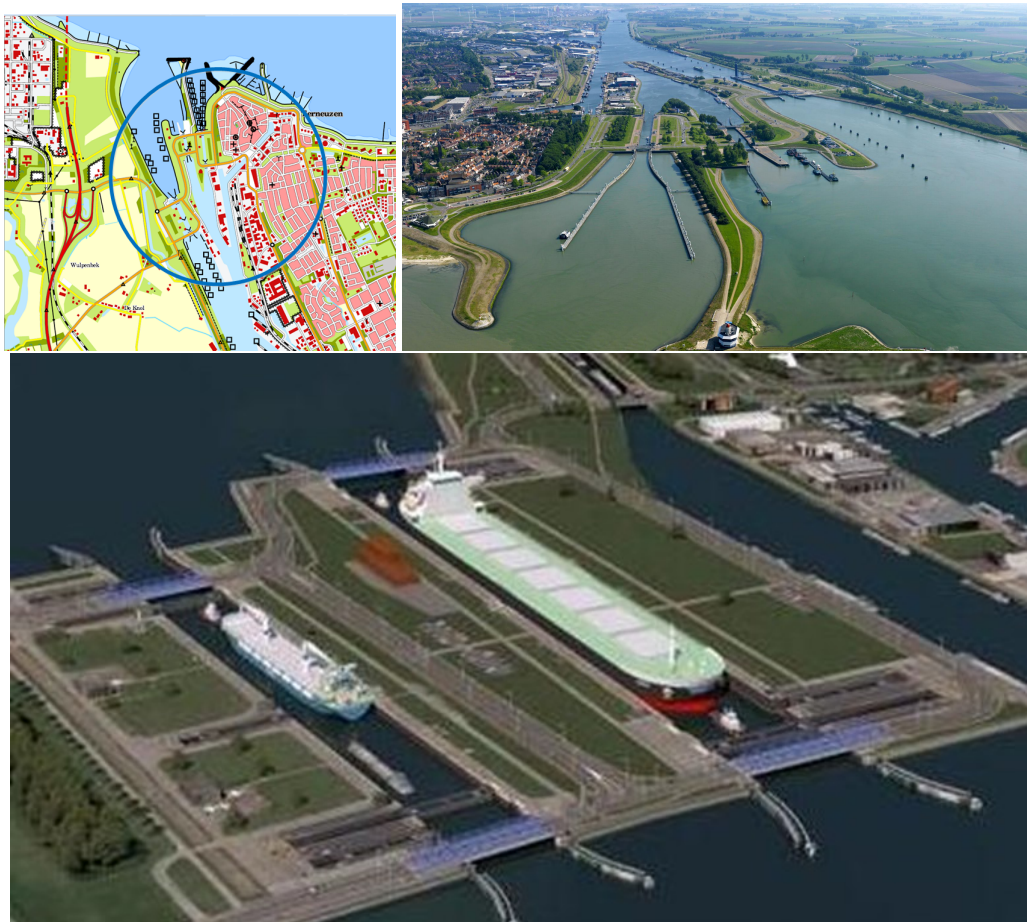
Figure 5.11: Location of the complex (upper left), an overview of existing complex (upper right), and an artist impression of the Terneuzen navigation lock complex after replacement of the Middensluis (bottom)
