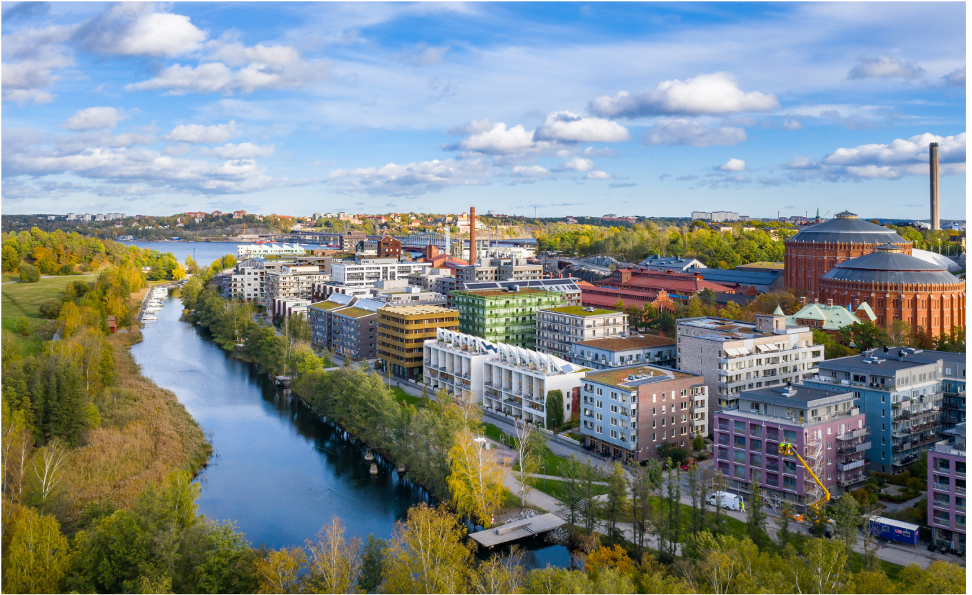
View on Husarviken, Hjorthagen and the two gasholders Source: Jansin & Hammarling/Stockholms Stad (2021)
