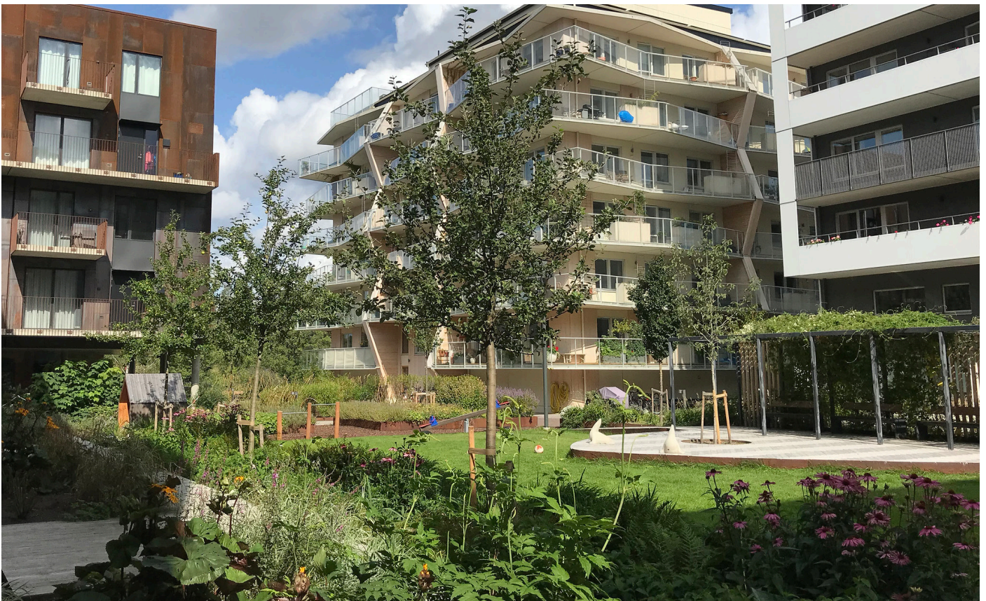
An example of one of the inner courtyards Source: Eva Nielsen/Stockholms Stad (2020)
