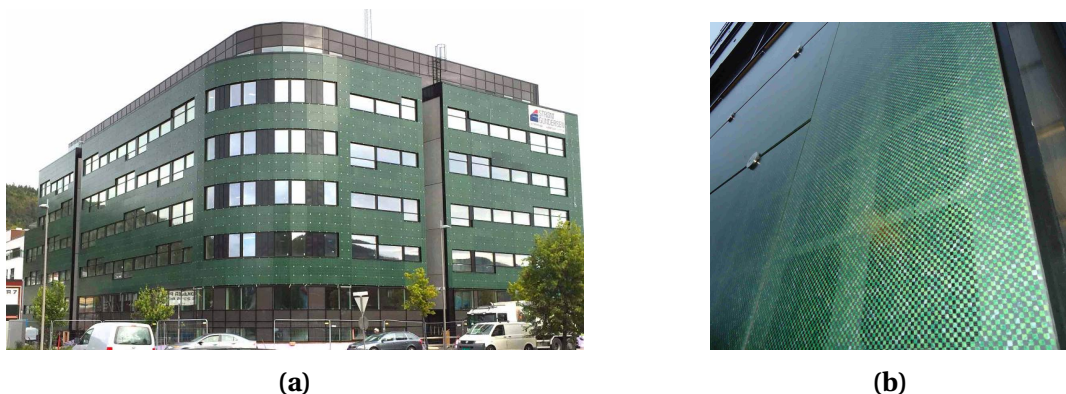
Figure 2.9: (a) Union Eiendomsutvikling Energy Building (Oslo, Norway). (b) Detail of the screen printed colored layer on the PV glass. Adapted from [22].
