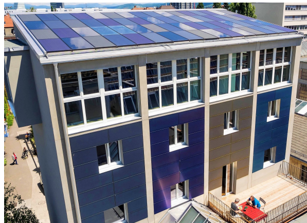
Figure 2.7: Coal silo building in Basel. Façades and roof covered by PV modules encapsulated with colored Kromatix™ glass. Adapted from [18].
