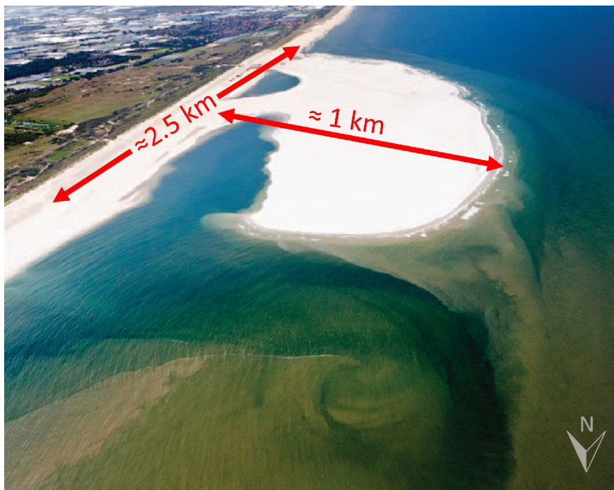
Figure 1: Aerial photograph of the Sand Motor after completion (September 2011). Note the clouds of fine-grained material moving to the North. Picture courtesy of Rijkswaterstaat / Joop van Houdt
