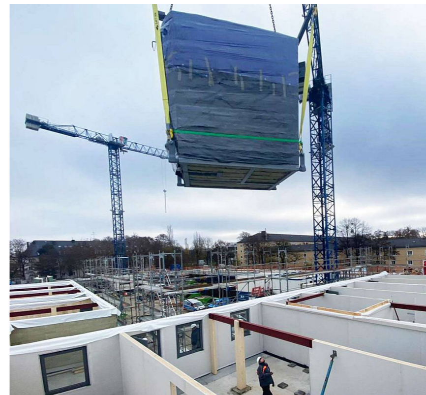
3D system W/C Module being lifted into place
