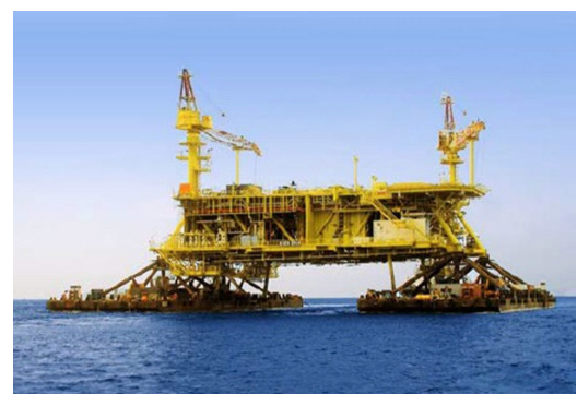
Figure 7.7: Dual vessel float over installation [63]
