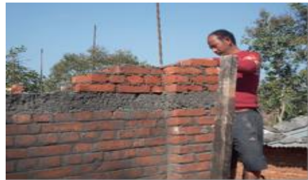
Figure 98: Construction on site
