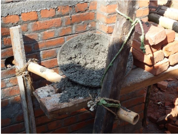
Figure 11: bucket used to measure volume proportions of components
