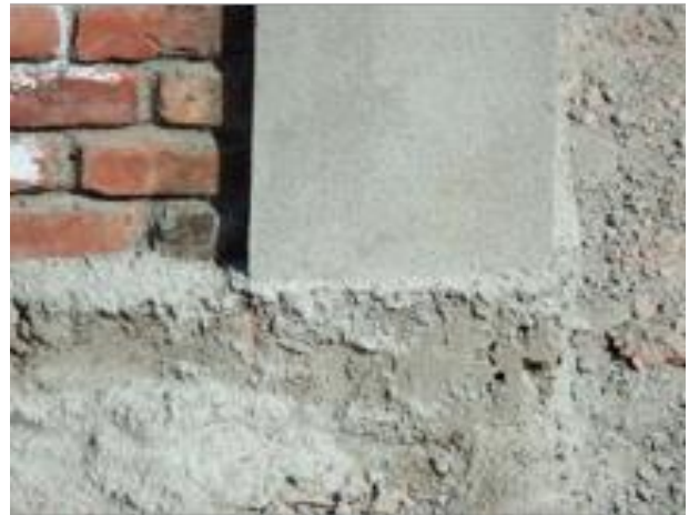
Figure 101: Concrete element with no planarity at the village of Ratankot
