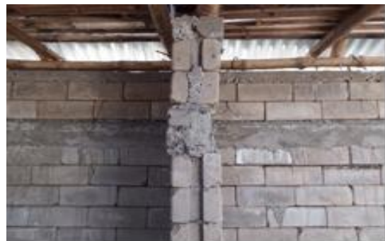
Figure 102: Concrete element with no planarity at the village of Ratankot
