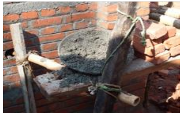
Figure 99: Construction on site
