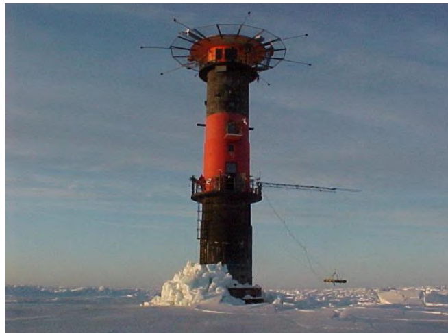
Figure 1.1: Photograph of the Norströmsgrund lighthouse, an exemplary offshore structure in the subarctic Gulf of Bothnia from Bjerkås et al. (2013).
