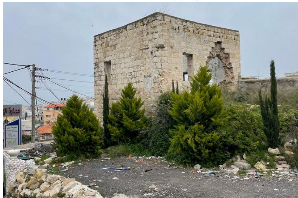
Photo 1: Overview on old building
