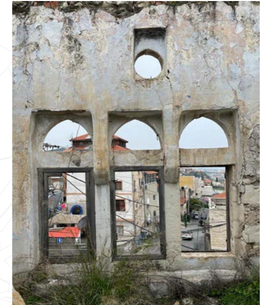
Photo 7: South view in the building
